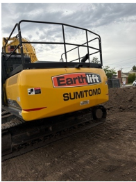
Rear of plant
